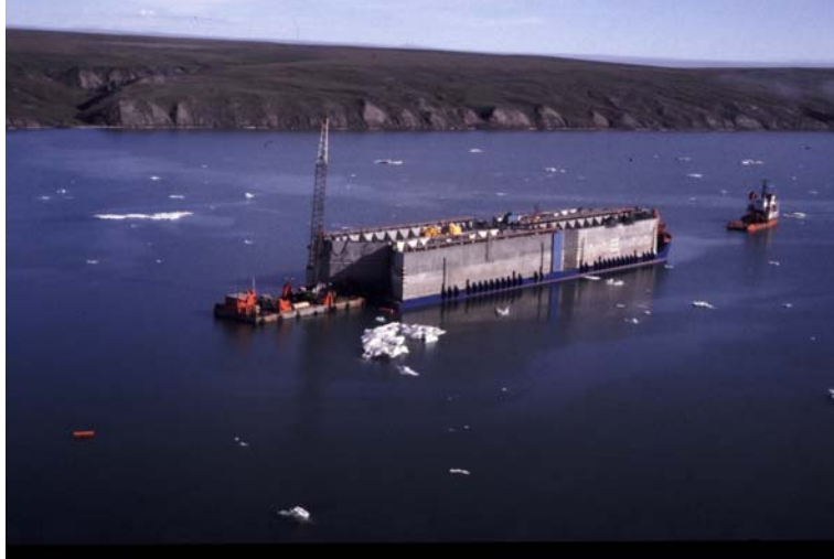
Figure 42. Transporting Concrete Caisson to Drilling Site
