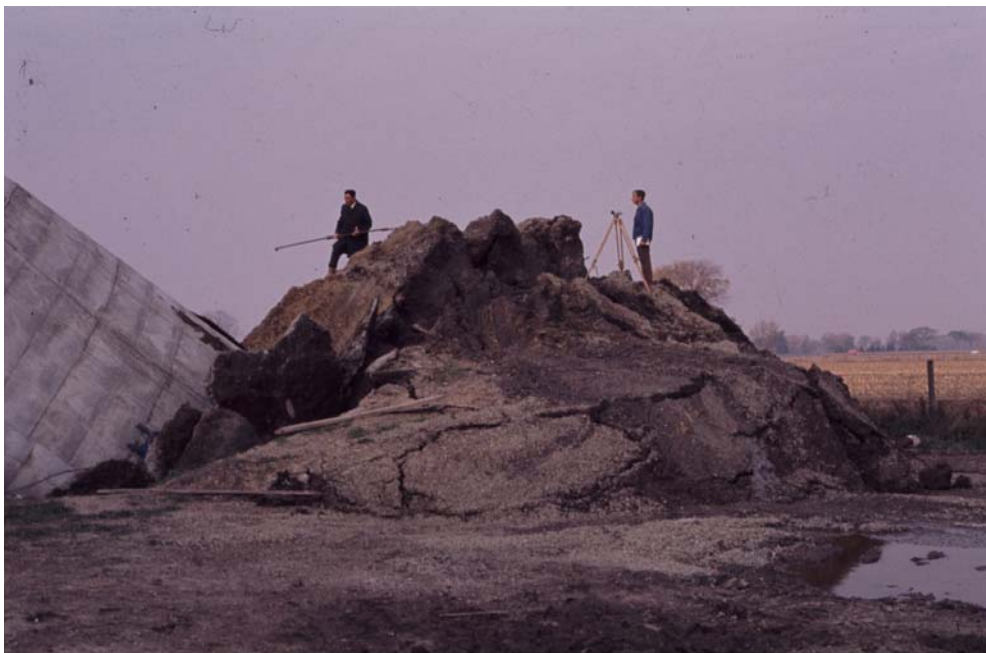
Figure 40. Heaved Foundation Soil due to Bearing Capacity Failure
