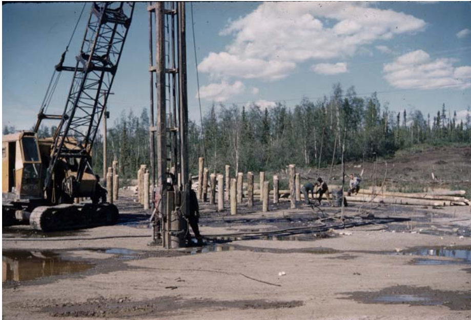
Figure 34. Installing Wood Piles in Permafrost
