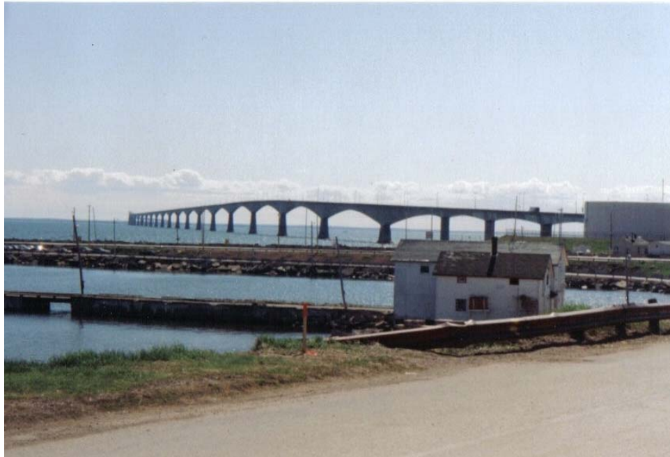
Figure 55. Confederation Bridge, 12.9 km Long
