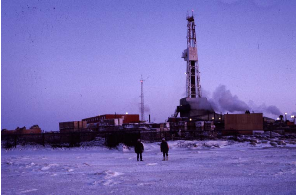
Figure 41. Oil Drilling from Artificial Island at Alerk, enclosed by Sea Ice in the Beaufort Sea
