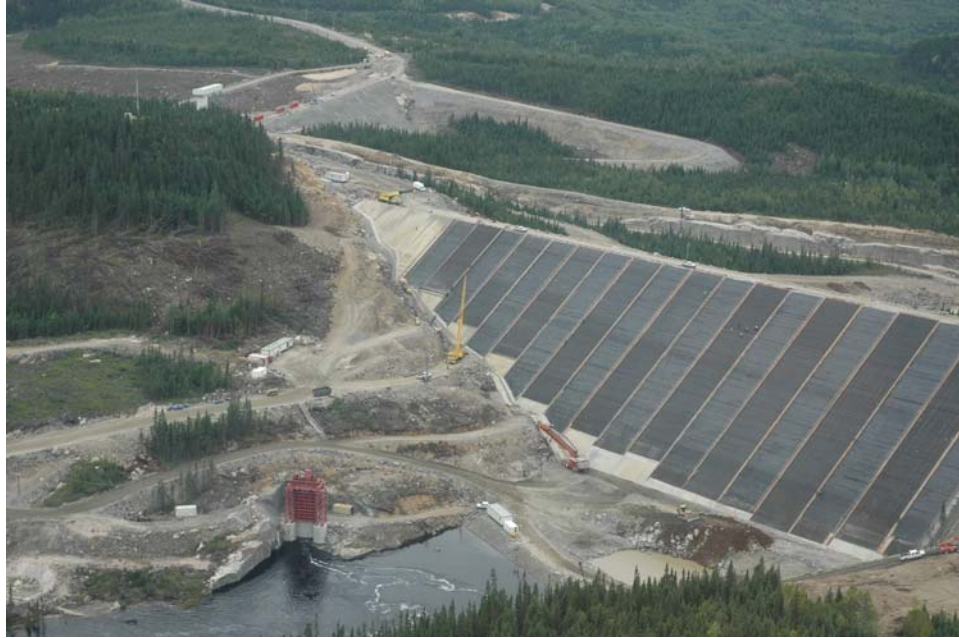
Figure 54. The Hydro Electric Power Development at Péribonka, Québec
