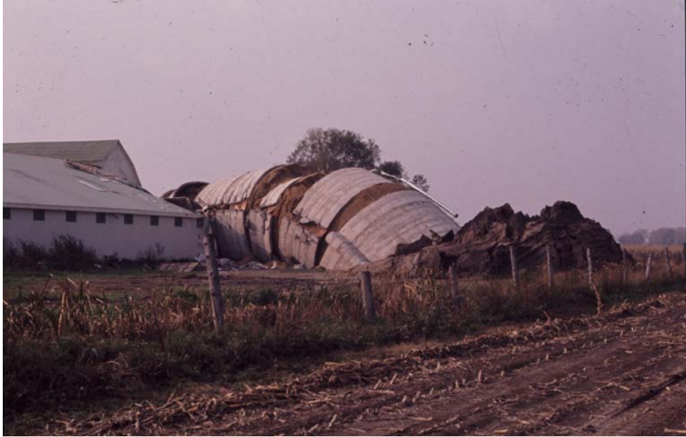
Figure 39. Bearing Capacity Failure of Farm Silo at Vankleek Hill, Ontario, 1970.
