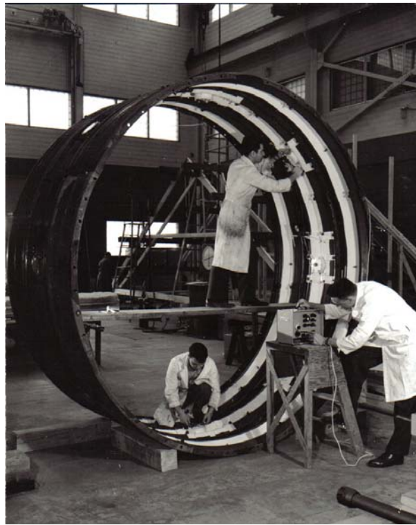
Figure 22. Instrumenting a Steel Tunnel Liner for the Ottawa Sewer Tunnel. Bill Eden, Michael Bozozuk and Lynn Boyd, 1956
