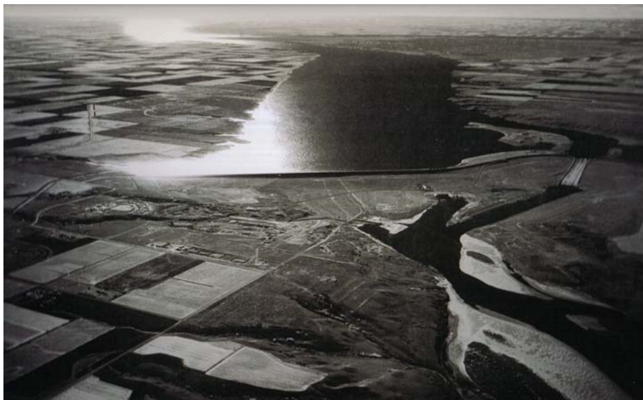
Figure 45. Gardner Dam and Lake Diefenbaker
