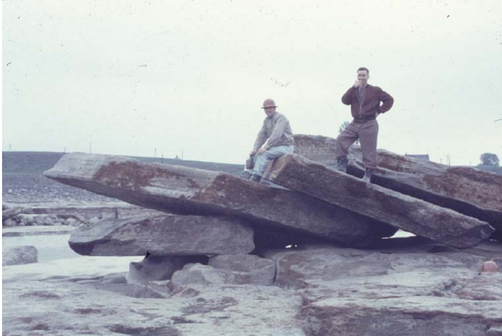
Figure 53. Dewatering Long Sault Rapids Revealed Huge Slabs of Dislodged Bedrock, Stacked Up Like Playing Cards
