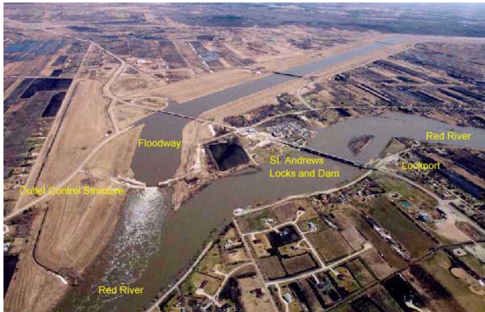
Figure 46. The Red River Floodway
