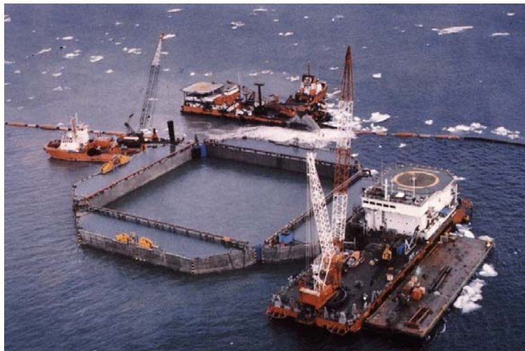
Figure 43. Assembly of Four Caissons over Submerged Sand Berm
