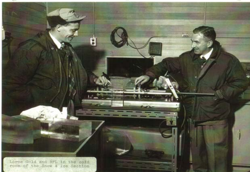
Figure 28. Lorne Gold (left) Demonstrating Trimming of Ice Specimens to Dr. Legget in the Cold Room, Snow & Ice Section of the Division of Building Research
