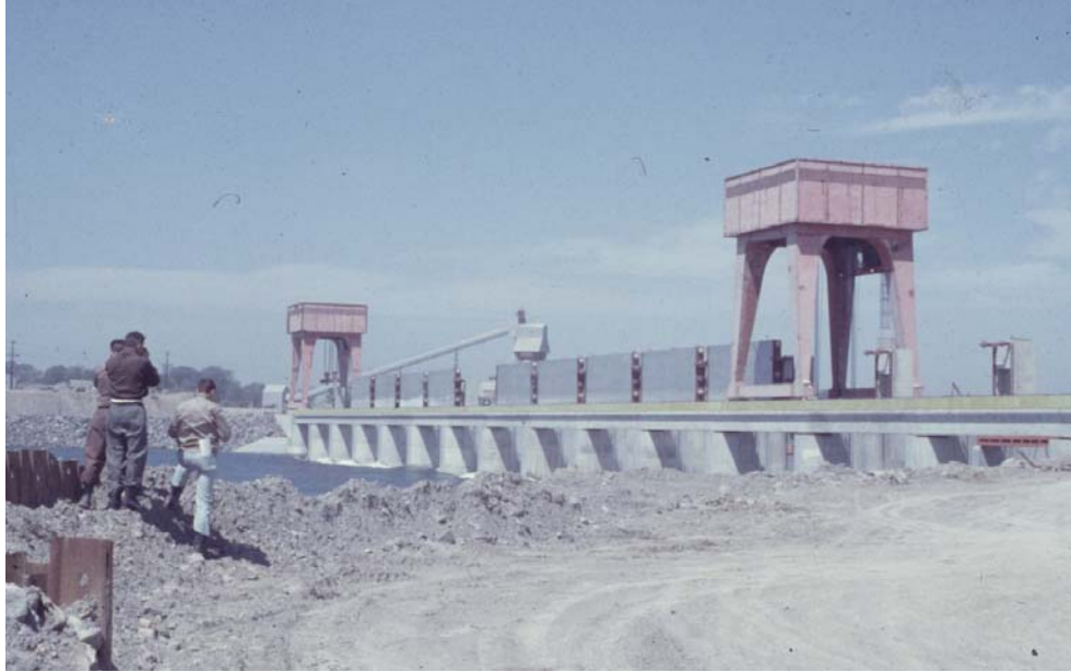
Figure 52. R.H. Saunders Dam, Height 53 m., Length 500 m., 1958
