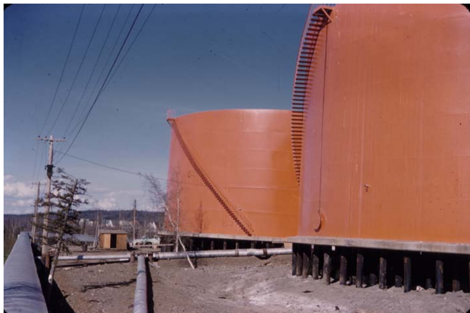
Figure 35. Heavy Oil Reservoir Supported On Wood Piles in Permafrost
